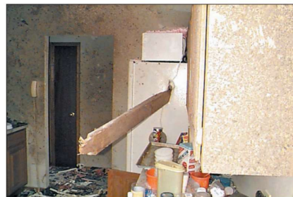
Figure B8-9. Refrigerator pierced by a 2x6. The portion of the 2x6 that is visible was 4 feet 8 inches long. It went several inches into the freezer compartment. (Oklahoma City, OK, 1999 tornado)
