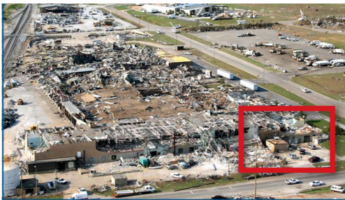
Figure 1: An EOC in Tuscaloosa, AL, that saw a loss of operations but remained intact even though the story above it collapsed (Tornado 2011)
