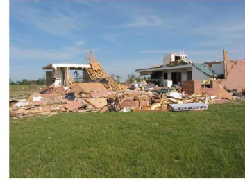
FR12: DOD 10: Total destruction of entire building
