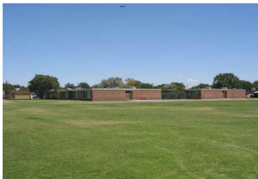
ES: Single story with flat roof; built-up roofing with gravel; brick veneer; large percentage of window glass; long interior hallways; load-bearing walls
