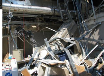
Interior following breach of envelope
