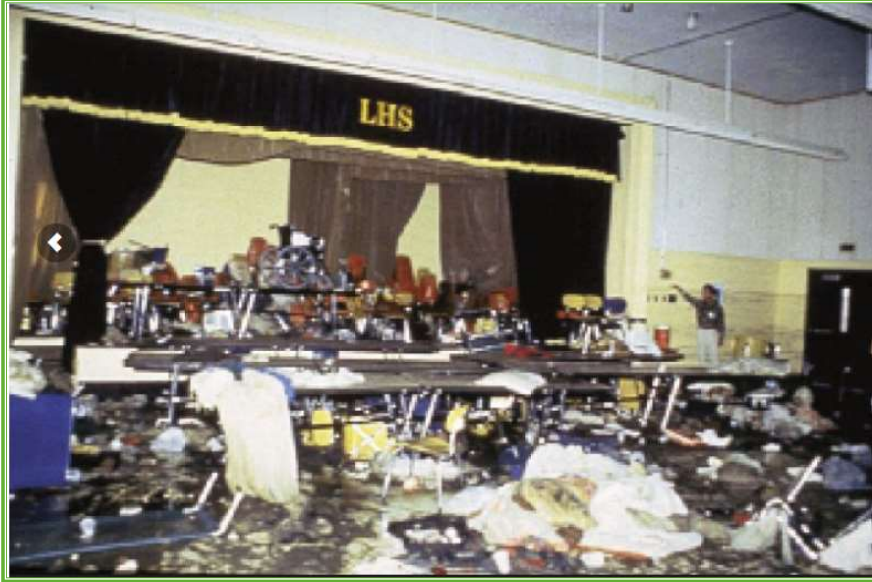
Lincoln High School McClennville SC Hurricane Hugo, 1989
