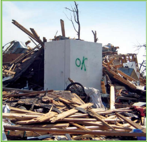
In-Residence Safe Room Joplin, MO, May 22, 2011
