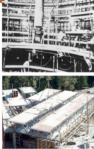
Slip forming of missile silo, Nov. 1960.
