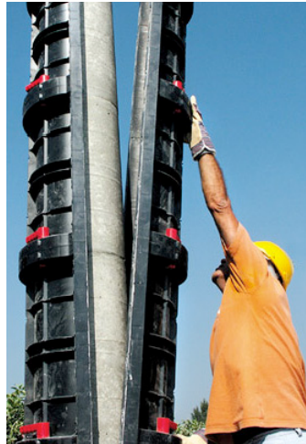
The "Geotube", a reusable plastic type of form.
