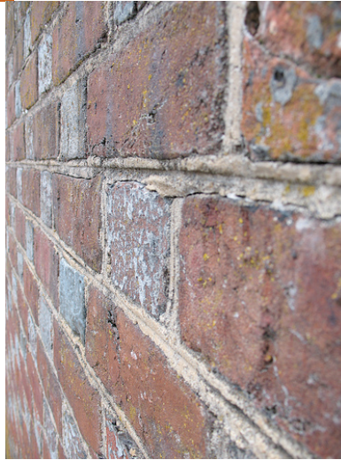
Flemish bond with glazed headers and struck joints. Stratford Hall, Westmoreland County, Virginia. Birthplace of R. E. Lee – Source: http://www.flickr.com/photos/3tuxedocats/2275792944/ , March 2008
