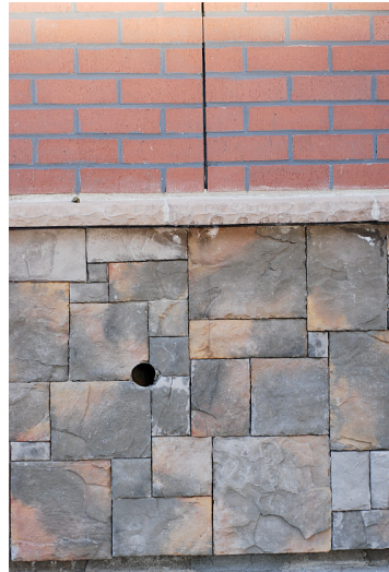
Fake brick on top of stone veneer used on exterior walls of Dog House Grill, Fresno CA – Image used only for application of expansion joint – NOT real Masonry
