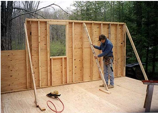
Sawn Timber Stud Walls
