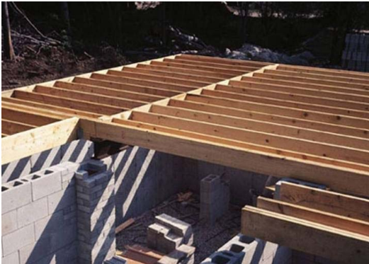
Sawn Timber Floor Joists
